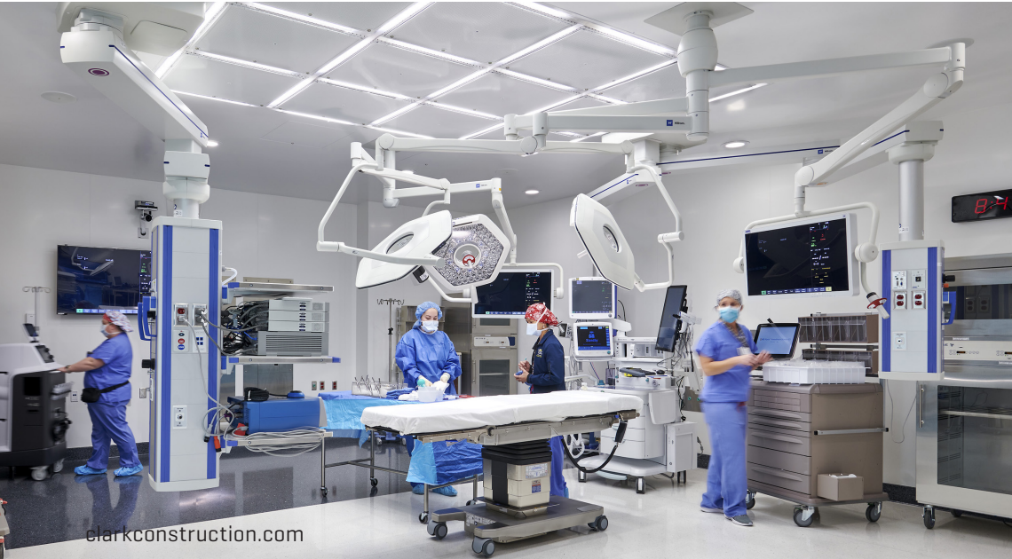
Prefabricated ceilings support future upgrades in medical technologies by containing steel infrastructure that accommodates maximum equipment needs, facilitating future installations of new operating room technology.
